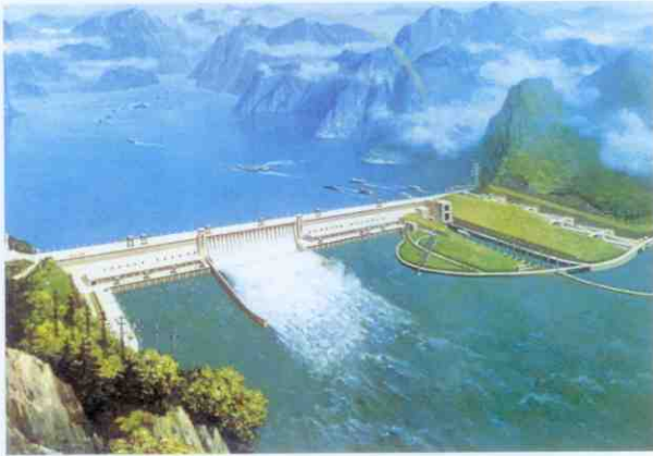
三峡水电站 Three Gorges Hydropower Station
