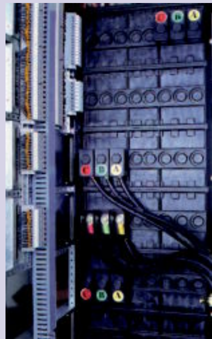
电缆和控制线连接(后出线) 图十三 Connecting of cable and control line (rear outgoing) Picture 13
